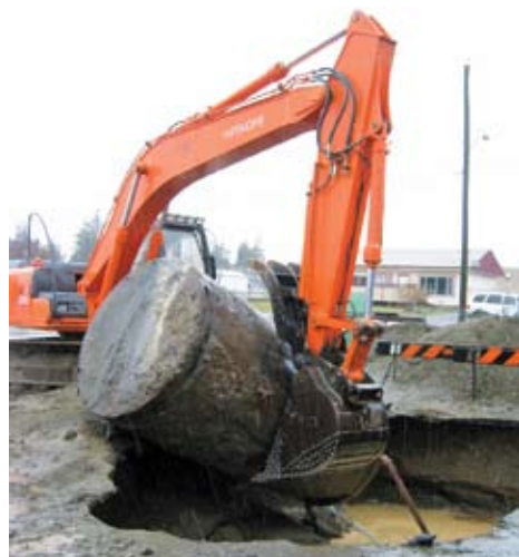
Underground storage tank removal – Wei Wai Kum First Nation.
