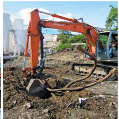
Fuel pipe removal – Heiltsuk First Nation.
